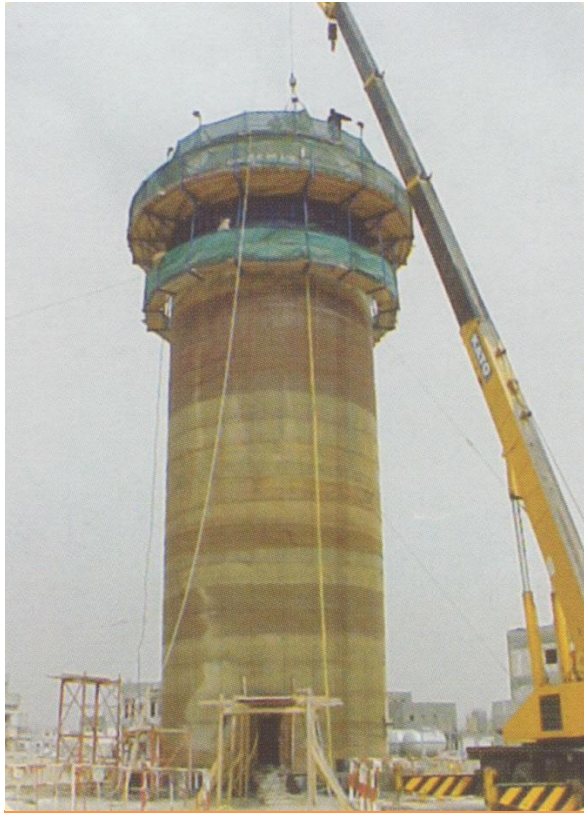
Slipforming of the structural support
