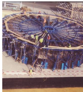
Tapered slipforming equipment during erection
