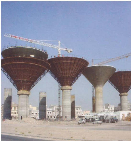
Using the form of basket for execution of the elevation tank at Jahra – Kuwait 2004
