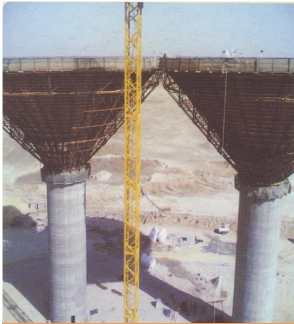
Execution of the tank using the form basket
