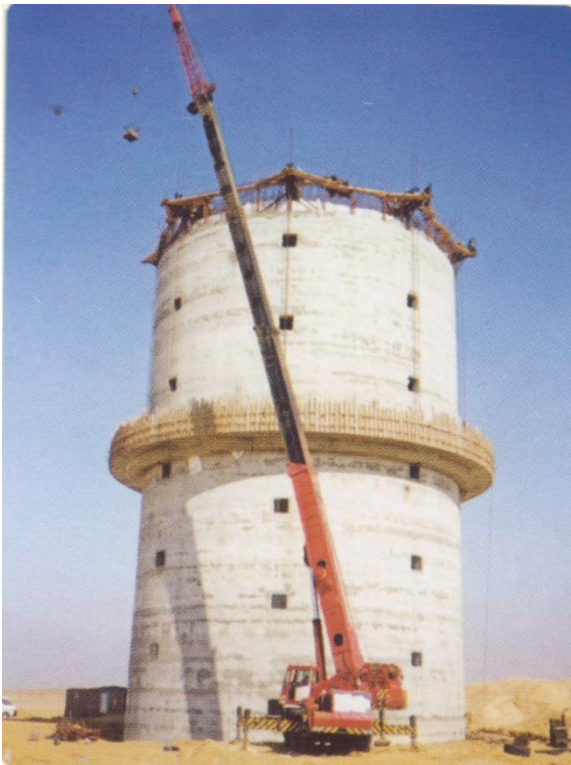
Lifting of the three slabs up to the level of tank bottom
