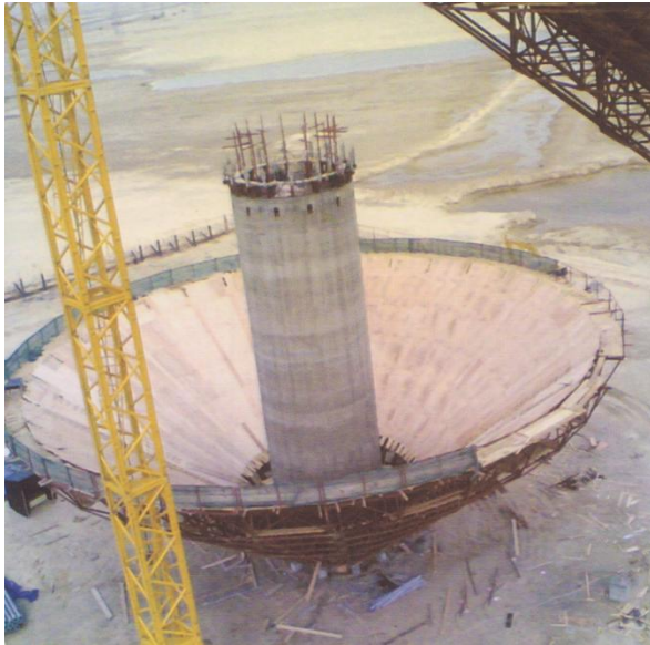
Using the form of basket for execution of the elevation tank at Jahra – Kuwait 2004
