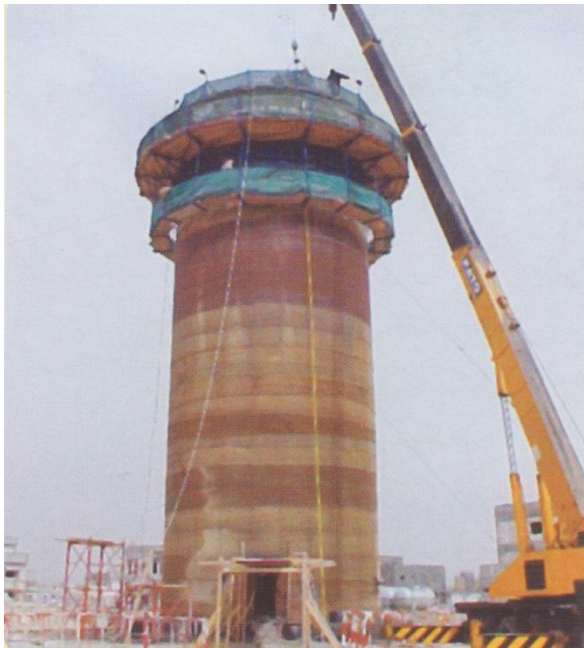
Slip forming of the structural support of the tank
