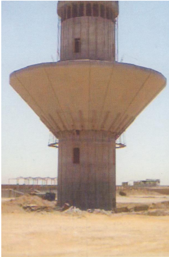
Tank during lifting operation
