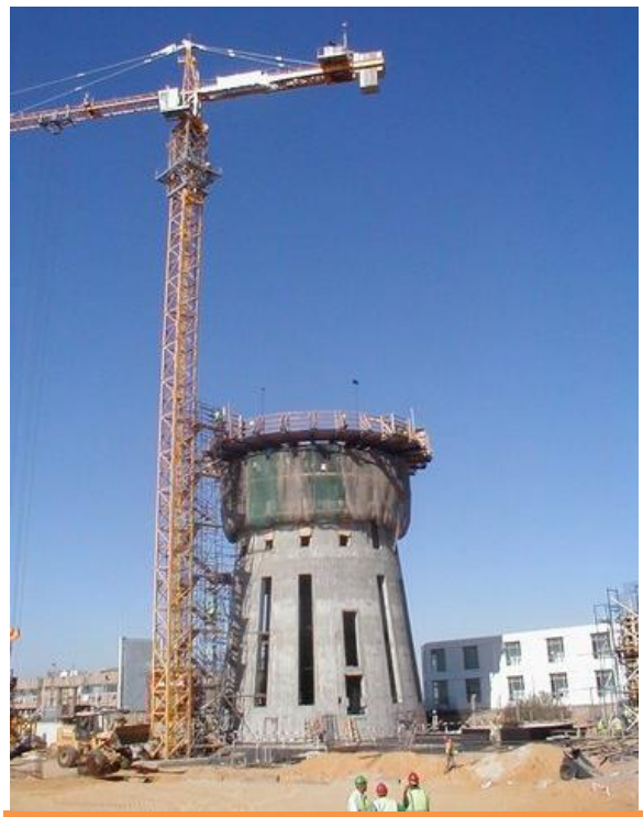
Slipforming of the structural support
