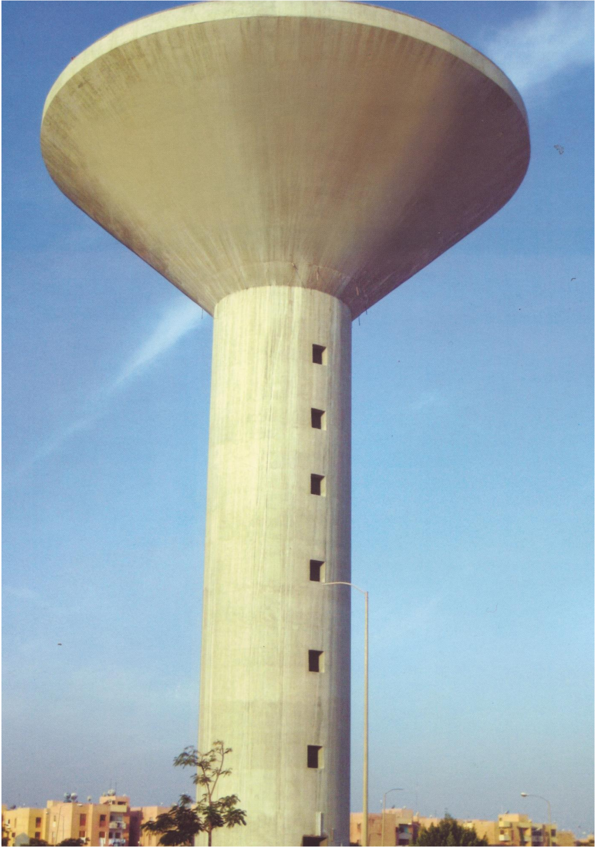
Elevated tank in their final shape (lifting of tank capacity 1760\text{m}^3 weight of the tank 2000 tons – at sadat city – 2006)
