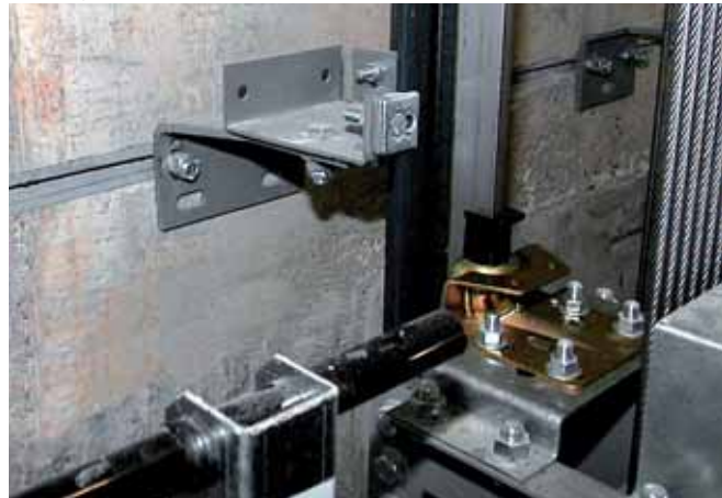
Fixing for guide rails
