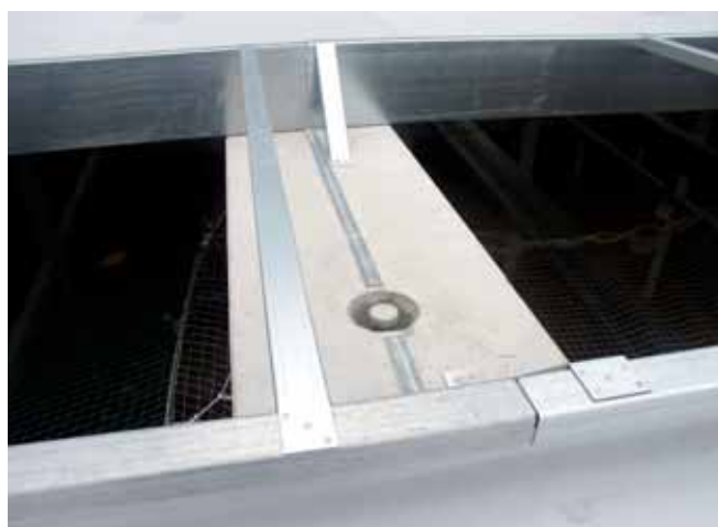
HALFEN HTU Cast-in channels in a prestressed concrete beam
