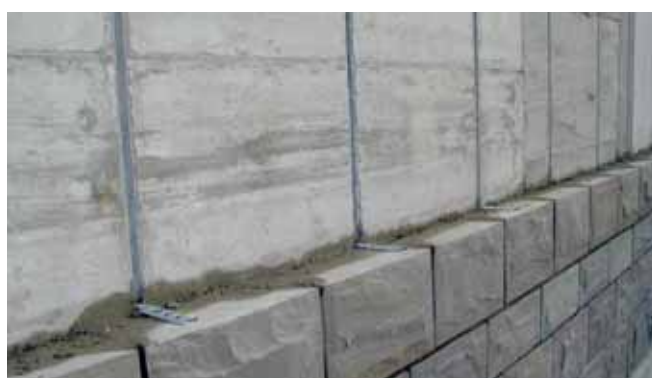
HALFEN ML Brick-ties anchor system
