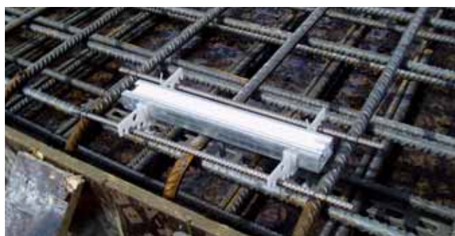
Installation with HALFEN ChanClip (see 2.2.2)
