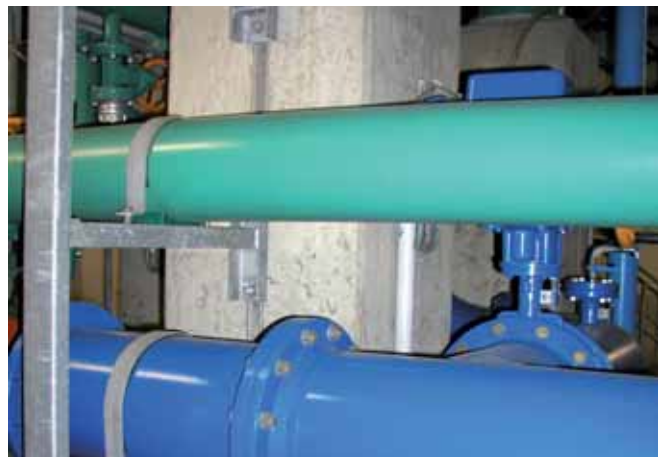
Pipe supports on vertical HZA-channels
