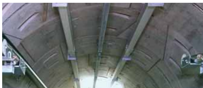
Curved HALFEN Cast-in channels in tunnel segments
