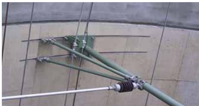
Fixing of over-head cables in railway tunnels
