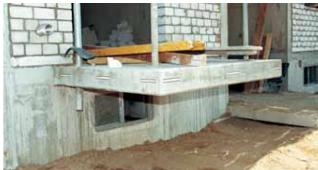
Cast-in HGB Channel, residential building
