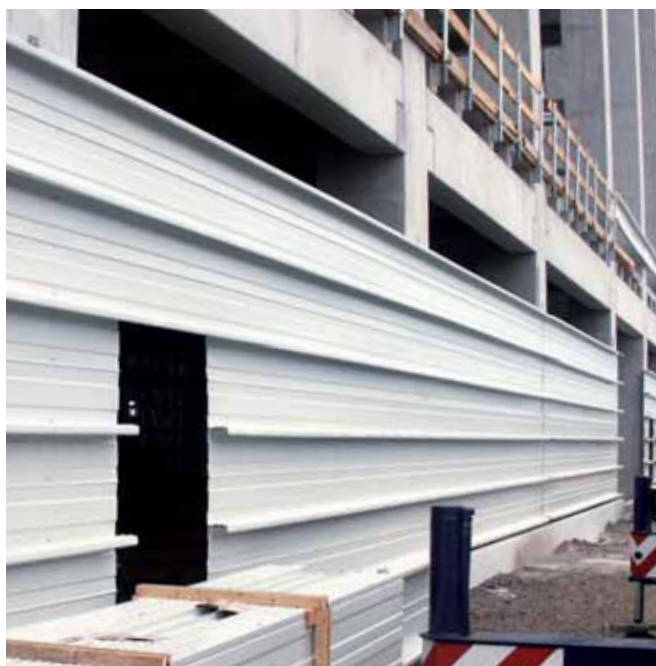
Façade fixed using HALFEN HTU Cast-in channels
