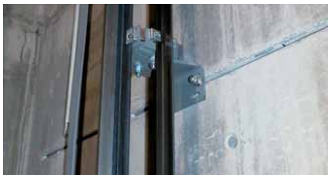
Fixing guide rails with HALFEN Channels
