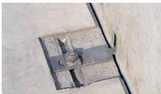
HALFEN HKZ Restraint tie with serrated washer
