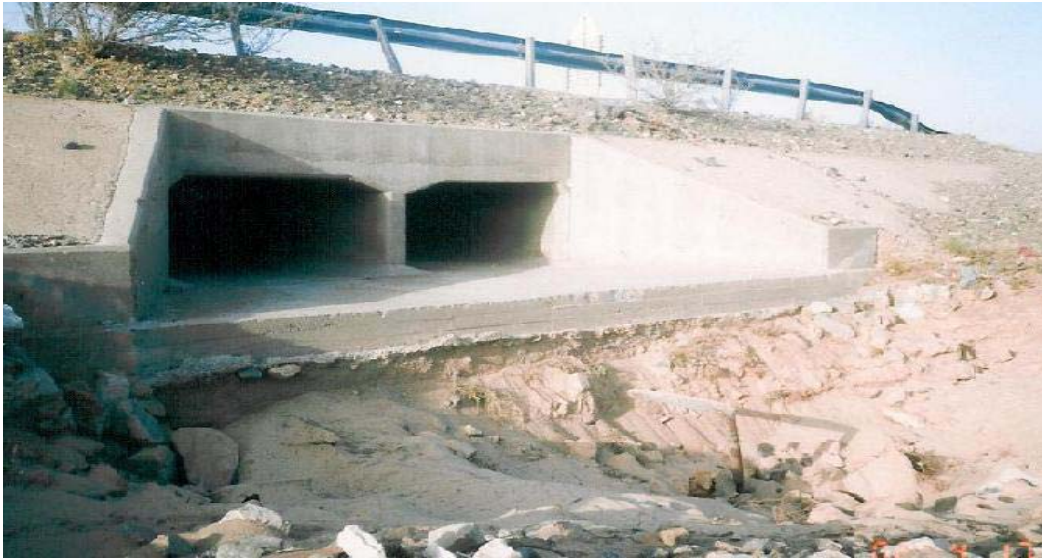
(Figure 3) A level of culvert higher than the level of ground surface. (Location: Makkah – Arafat road no.2)
