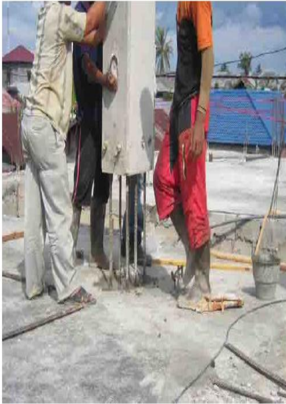
Figure 15. Precast column with ducting inside
