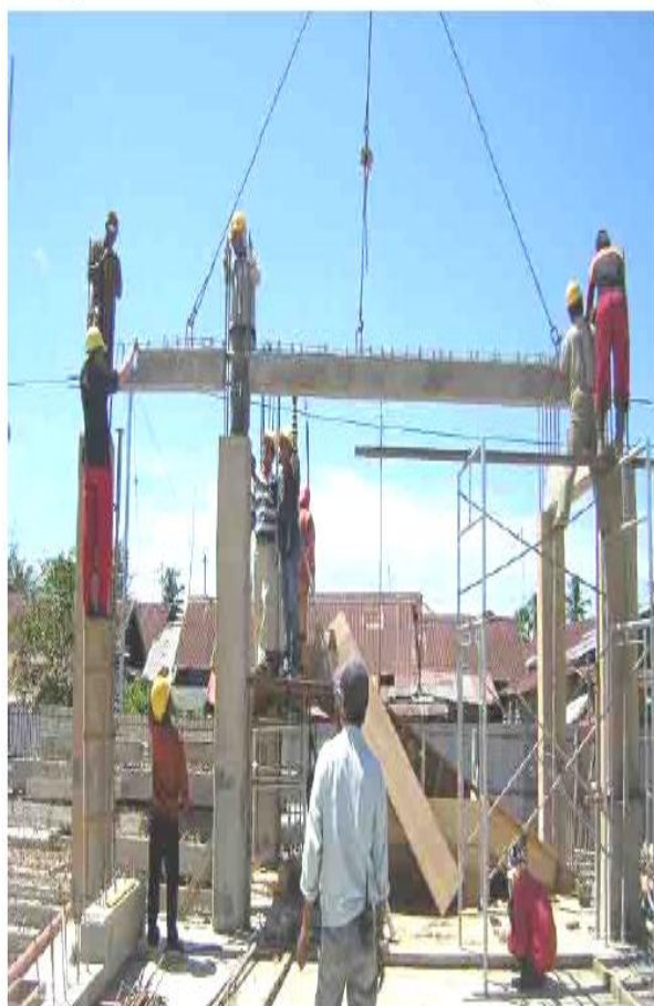
Figure 17. Erection of precast beams [5]
