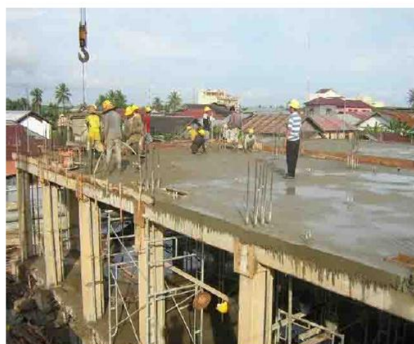
Figure 20. Concrete pouring for the top slab [5]
