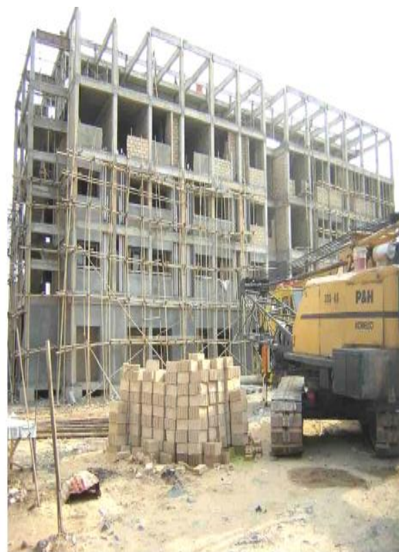
Figure 24. Completion of the full structural frames
