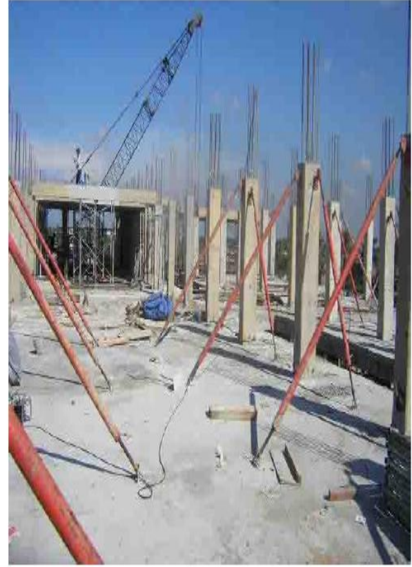
Figure 16. Precast columns after erection [5]
