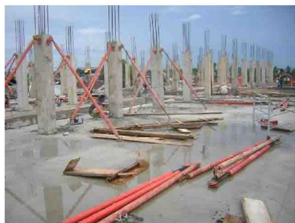
Figure 22. Prefabricated columns on 2 nd floor [5]
