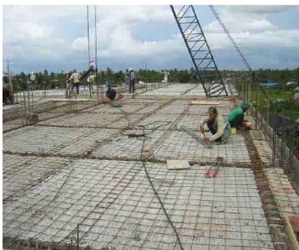
Figure 19. Wire mesh after precast half slabs
