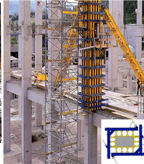
Column Formwork
