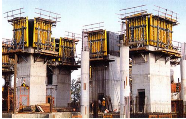
Lift Core Formwork
