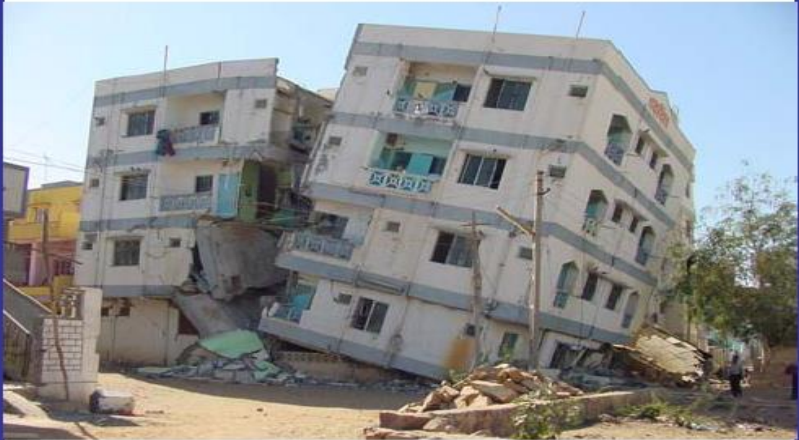
(b) Collapse of reinforced concrete columns (and building) during 2001 Bhuj (India) earthquake
