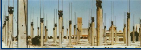
Used of 56 lifting jacks to lift hall no.3 Cairo airport
