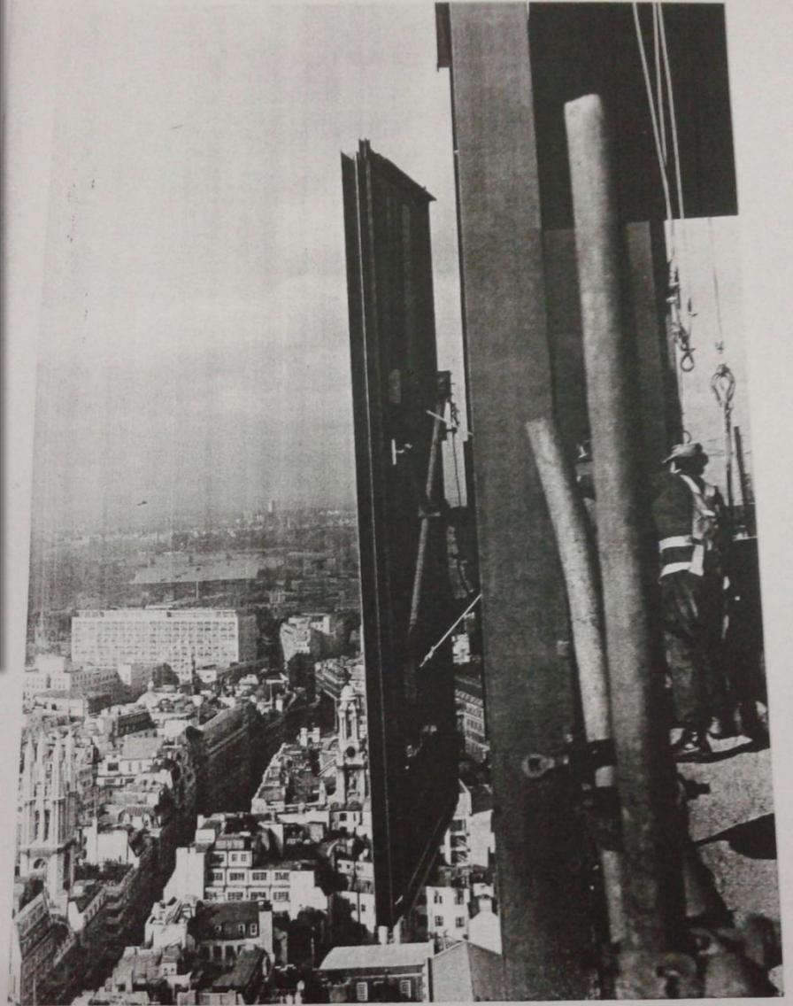
Fig. 15.10 Glazing of Commercial Union building. Glazed frame turned and ready to be brought back into fixing position
