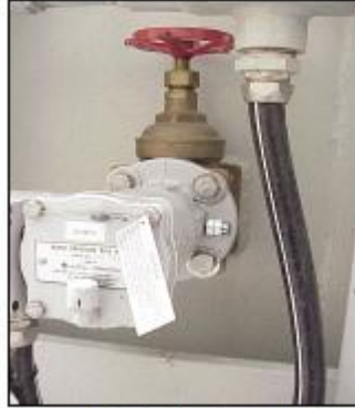
شكل 3-15 : Sudden Pressure Relay
