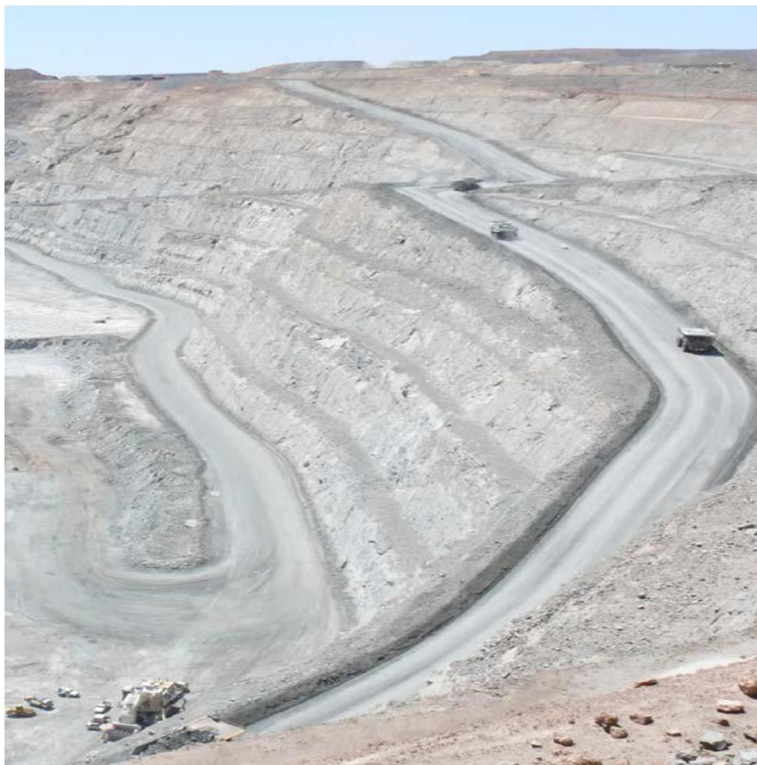
**Photograph 9 Haul road design and ramp gradients; on mining site.**
