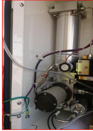
Pump & Injector unit
